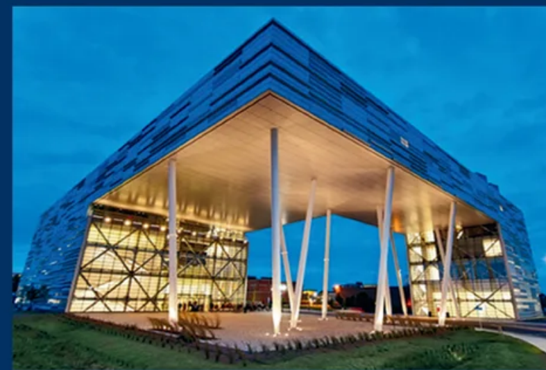
Rutgers University Business School Centralized Geothermal System Piscataway, NJ
