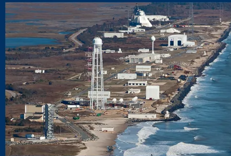
NASA Wallops Flight Facility Multi-Building and Centralized Campus Geothermal Systems Wallops Island, VA
