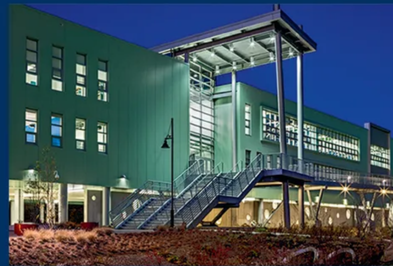
Marine Science Magnet High School Centralized Geothermal System Groton, CT
