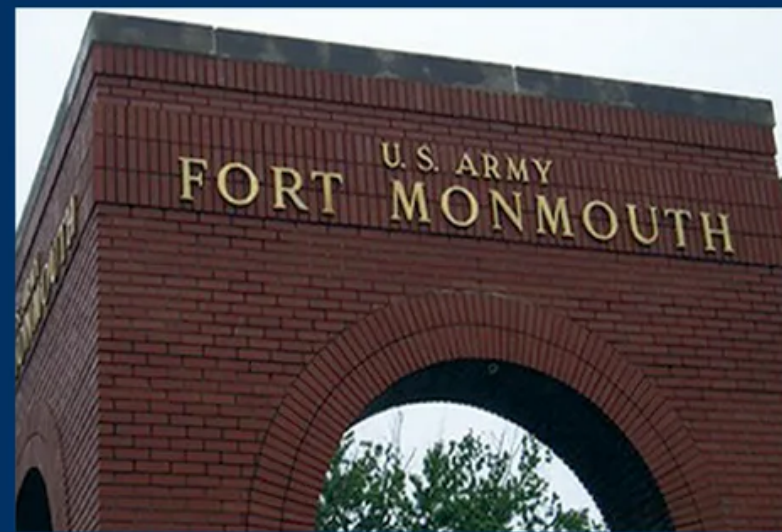
Fort Monmouth Army Base Multi-Building and Centralized Campus Geothermal Systems Eatontown, NJ
